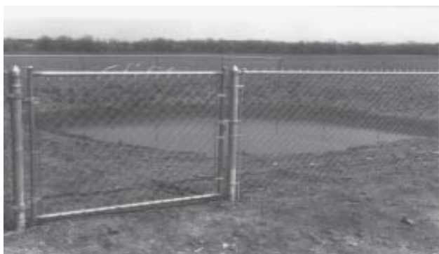
Figure 3. A well-constructed new wastewater pond — this chain-link fence will have a long life and requires little maintenance.
